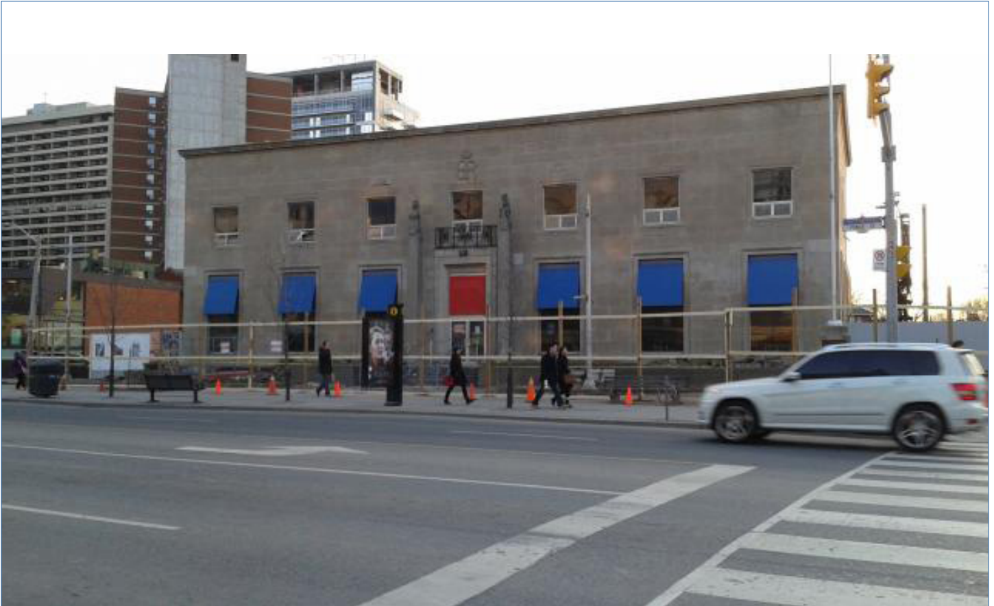
View of Postal Station K's Art Deco facade, image by UrbanToronto Forum contributor Roundabout
